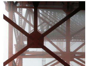
Golden Gate Bridge
