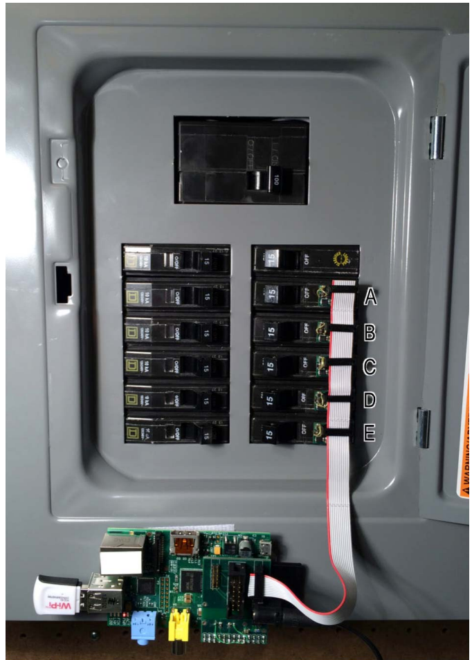
Fig. 3. PASEM system installation on circuit breaker panel. Five PASEM devices installed with wireless base station at bottom. Circuit breakers labeled for reference.
