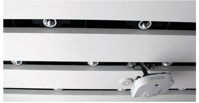
Figure 3: Recessed ceiling lights. Lights such as these are traditionally difficult to meter due to limited access to their wiring and uncertainty about the topology of the lighting circuit. Our Gecko sensors are easily and unobtrusively installed in fixtures such as these. See Figure 2(c) for a closeup view of the sensor mounting.
