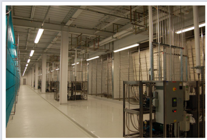
Evaporative cooling / humidification corridor
