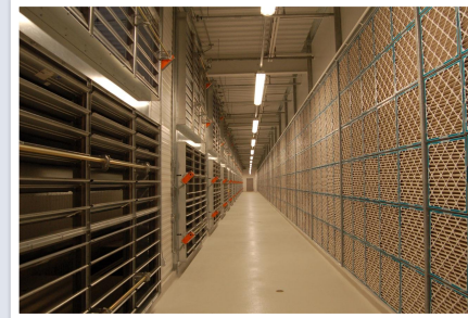
Air mixing section - Return air / out side air / filter corridor
