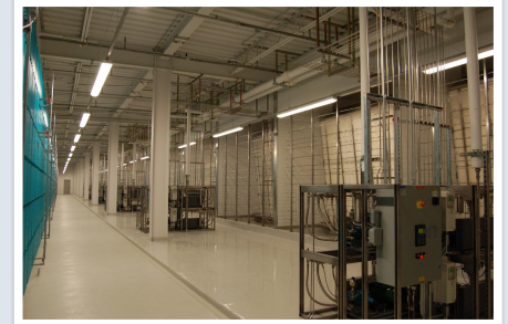
Evaporative cooling / humidification corridor
