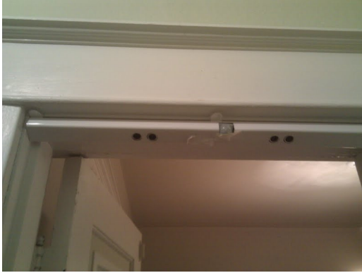
Figure 1. The doorway sensor is discretely mounted behind the door jamb in a molded plastic enclosure.
